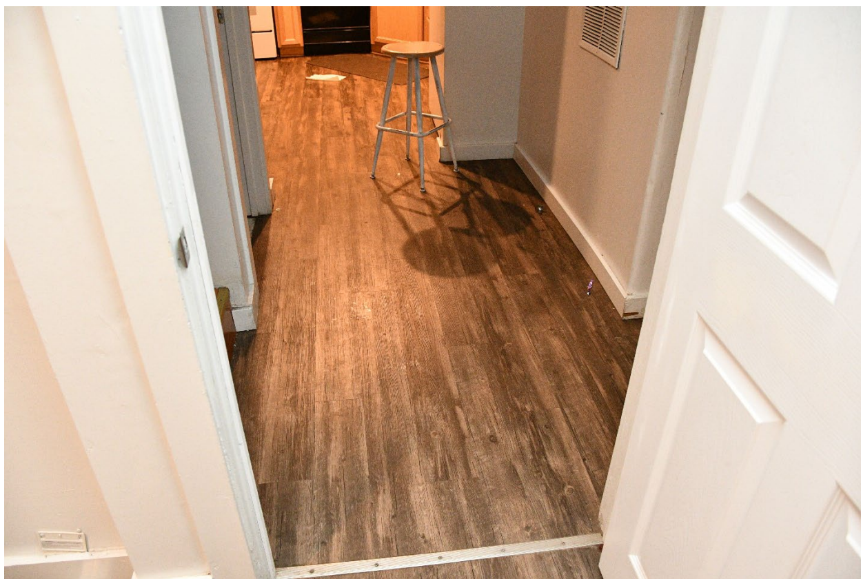
Looking Out the Door of D.M.'s Room, Photo 1, Taken 11.13.22 (File Name: ISP_4783.JPG)
